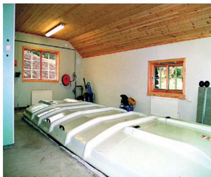
(Above) BK NuDisc® installed at a Youth Hostel in Norway to treat wastewater to a high degree including nutrient removal (phosphorus reduction down to under 1 mg/l). During Winter this 150 PE Plant treats wastewater from the Caretaker's family of 4 persons only, but in Summer the population can increase to 150 persons and for a short period of 4 to 5 weeks the population peaks to about 200 persons. This plant is installed in a building due to the extreme cold weather in Norway.
