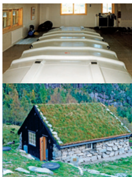
(Above) BK NuDisc® installed at a Youth Hostel in Norway to treat wastewater to a high degree including nutrient removal (phosphorus reduction down to under 1 mg/l). During Winter this 150 PE Plant treats wastewater from the Caretaker's family of 4 persons only, but in Summer the population can increase to 150 persons and for a short period of 4 to 5 weeks the population peaks to about 200 persons. This plant is installed in a building due to the extreme cold weather in Norway.
